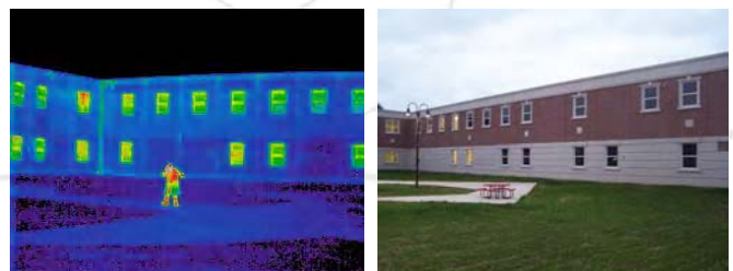
Figure 3: Courtyard – Thermal Image
