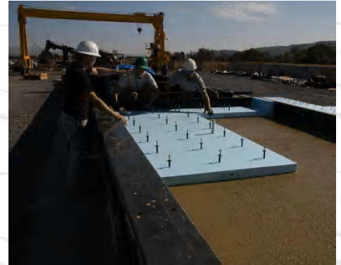
Figure 1: High Performance Panel Casting
