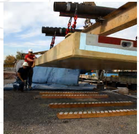
Figure 2: Sandwich Panel Off-loading
